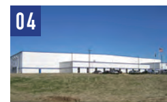
American Howa Kentucky, Inc. Georgetown Plant
