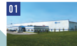
American Howa Kentucky, Inc. Kentucky Plant
